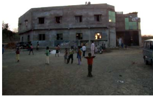
Front View of Building
